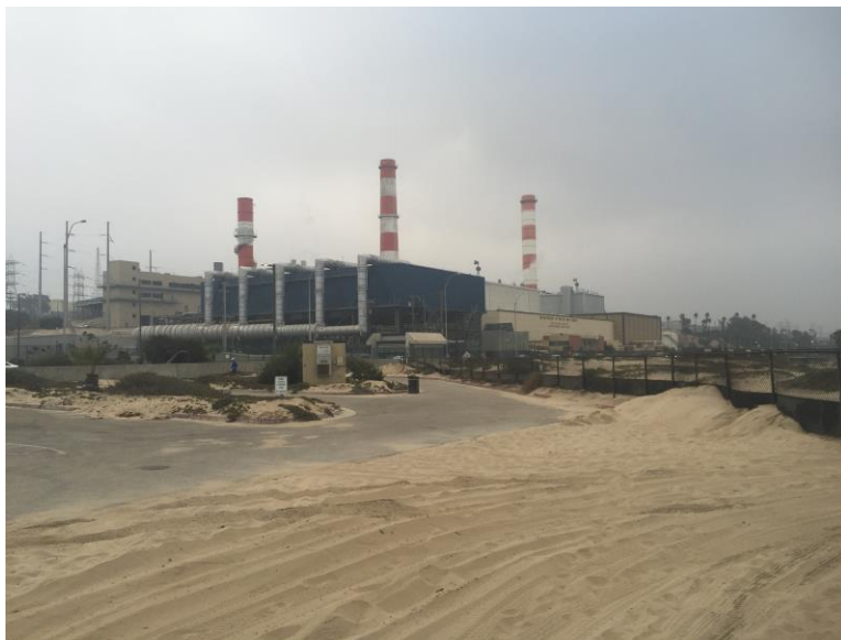
Photo 6: Department of Water and Power, Scattergood Steam Plant Looking South
