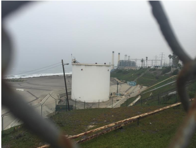
Photo 1: Chevron Storage, South of NRG Energy, Looking North
