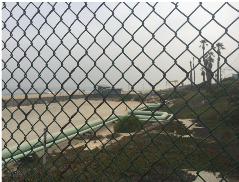
Photo 2: North side of NRG Energy meets South end of Dockweiler State Beach Looking North
