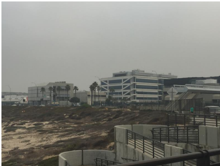
Photo 16: Hyperion Water Reclamation Plant, From Dockweiler Community Center Looking North East
